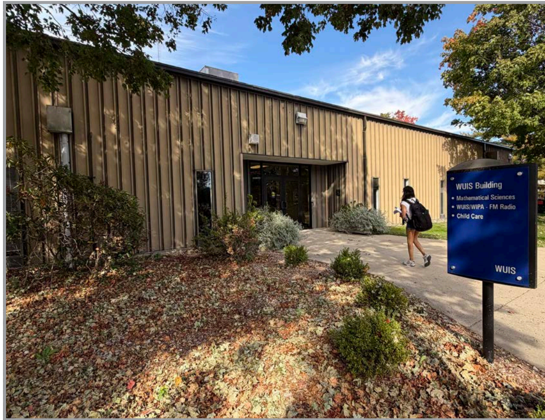
The WUIS building on the University of Illinois Springfield campus, shown here on Oct. 13, is scheduled to be torn down after the building permanently closes on July 30. PHOTO BY DEAN OLSEN
