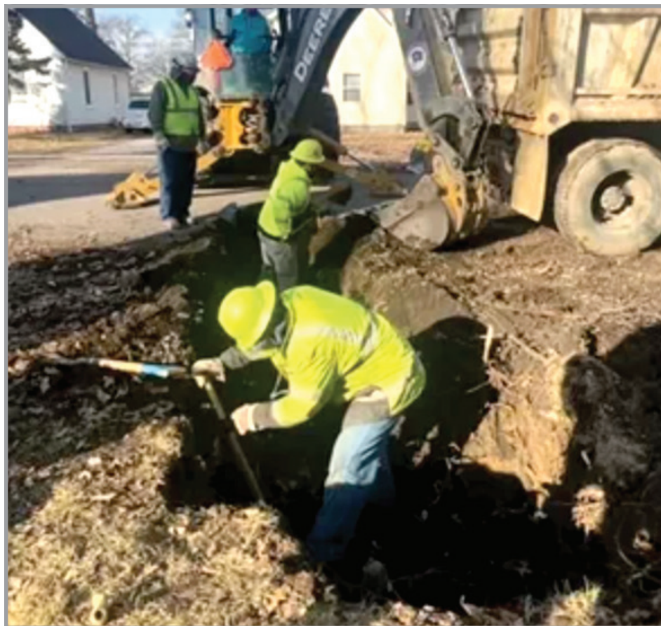
CWLP crews are working to remove the nearly 9,000 remaining lead pipes buried under Springfield's roadways.. PHOTO CREDIT CWLP.
