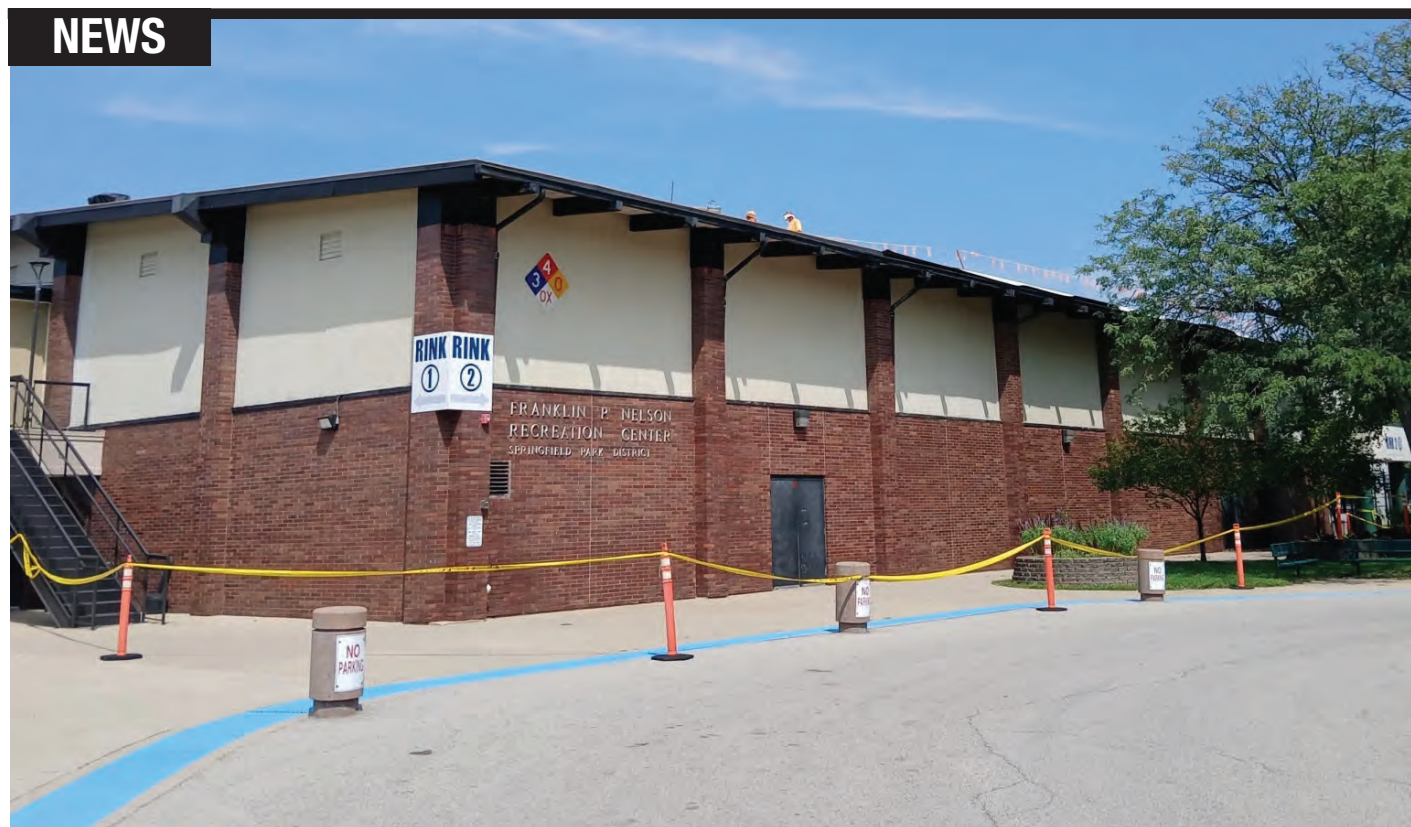
Workers lay on coating as part of the construction of the new roof at Nelson Center on Aug. 25. CREDIT: PHOTO BY MARIA GARDNER LARA
