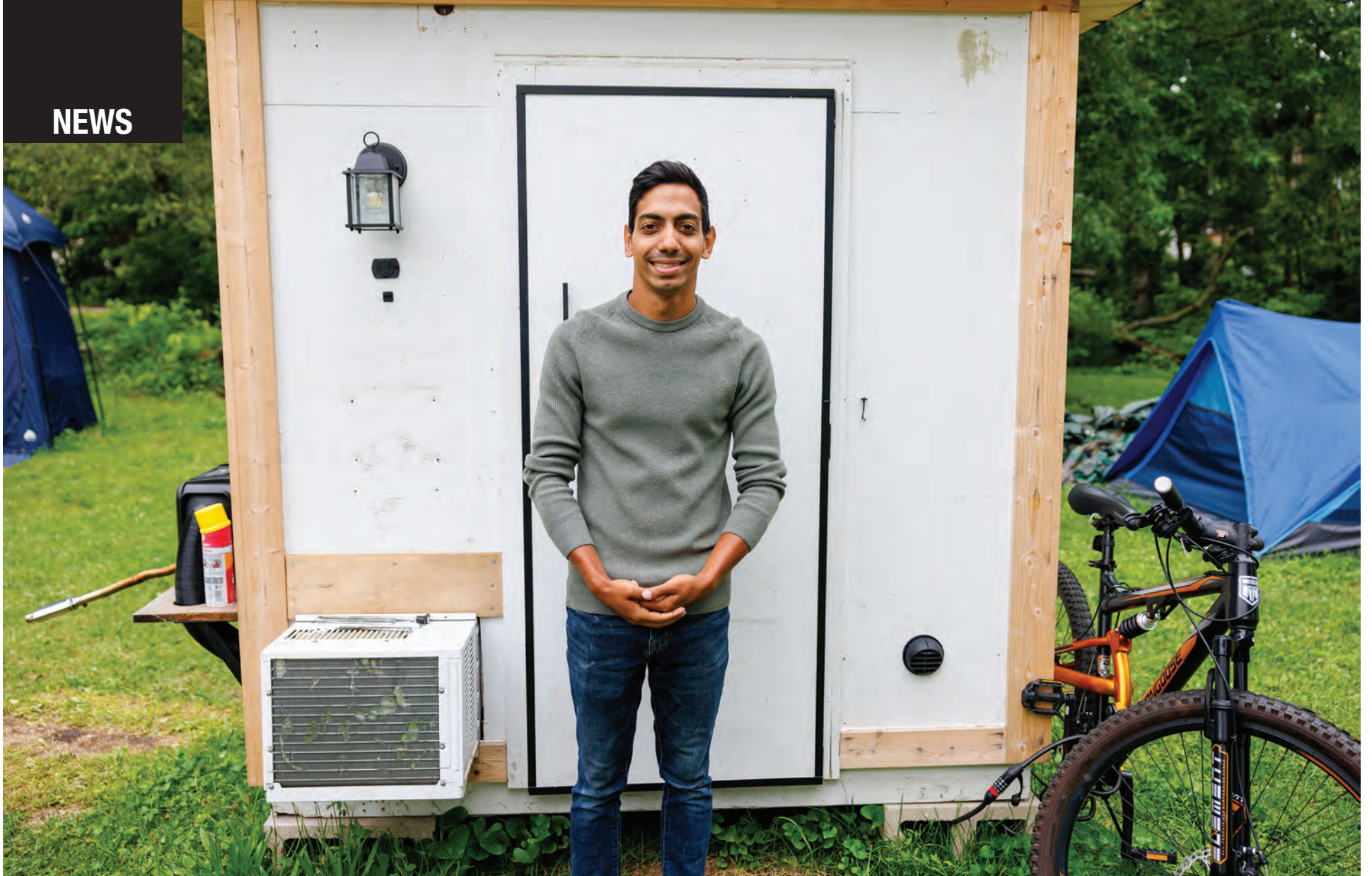
Chase Hadez, who goes by Colton Lexus, in front of his 18-square-foot home he built on a lot he owns at 17th and Carpenter streets. The city has ordered him to vacate it, saying it doesn't meet building codes or zoning requirements. PHOTO BY ZACH ADAMS
