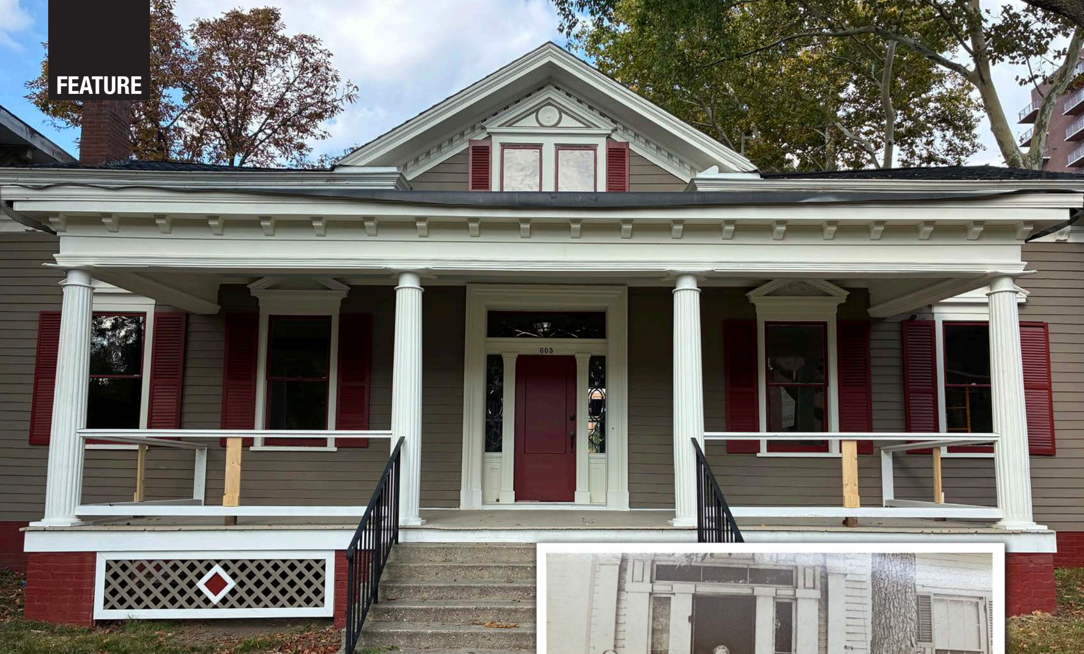
The porch-in-progress awaits railing balusters and column capitals.
