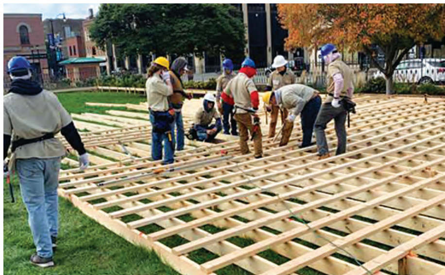
Capital Area Career Center building trades students building the platform.
