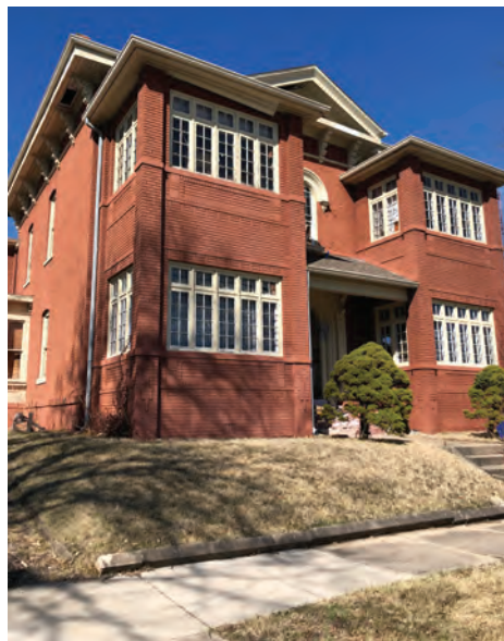
Wohlgemuth's residence, built in 1865, still stands at Eighth and Cook.
