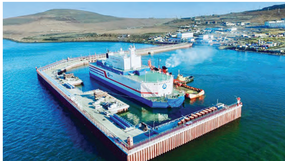
A barge next to the Russian city of Vilyuchinsk holds two Small Modular Nuclear Reactors which provide electricity for the town. It is one of two SMNR powerplants in the world. PHOTO BY ROSENERGATOM
