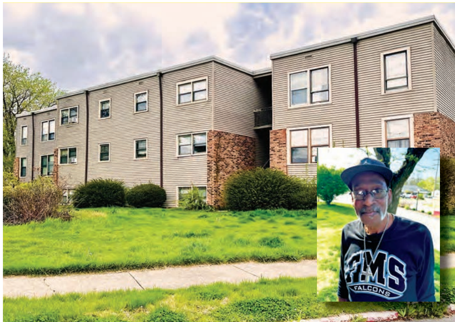
The New York investors who own Olde Towne Apartments are more than $100,000 behind on water and electric bills, and the city of Springfield has said CWLP will shut off service May 1, displacing the remaining tenants, if the past utility bills are not paid. PHOTO BY BRANDON TURLEY Right: Dennis Hull, a cafeteria worker for Springfield Public Schools, has lived at Olde Towne Apartments for 18 years and said he's never been behind on his rent. PHOTO BY SCOTT REEDER
